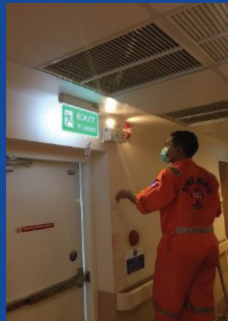
Fire Alarm System Testing (Smoke Detector, Heat Detector and Manual Station)
