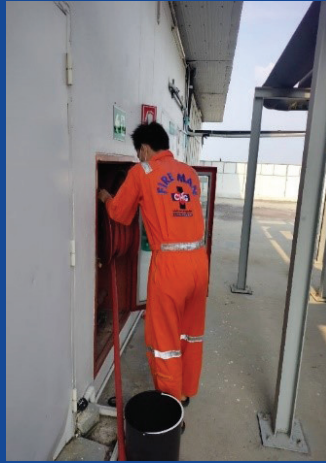
Fire hose and water supply Testing
