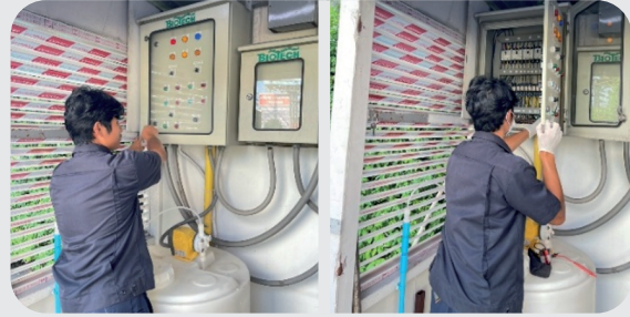
Inspection of aeration system control panels within wastewater treatment facilities
